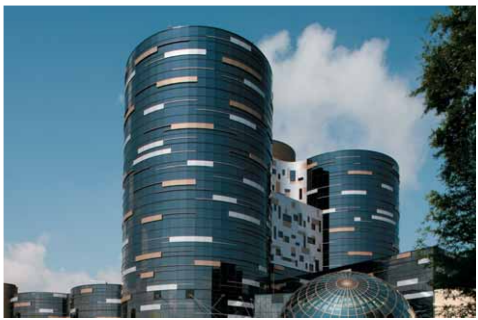
Winnie Palmer Hospital for Women & Babies Orlando, Florida Architect: Jonathon Bailey Associates Glazing Contractor: Harmon, Inc. Photographer: Bob Braun Photography
